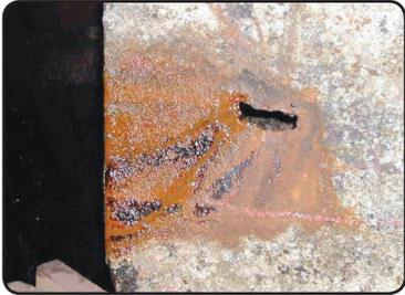
Mapping the extent and severity of individual pits by way of systematically checking pitting corrosion in each bay.
